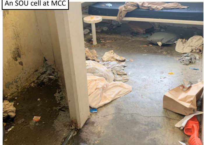
An SOU cell at MCC
